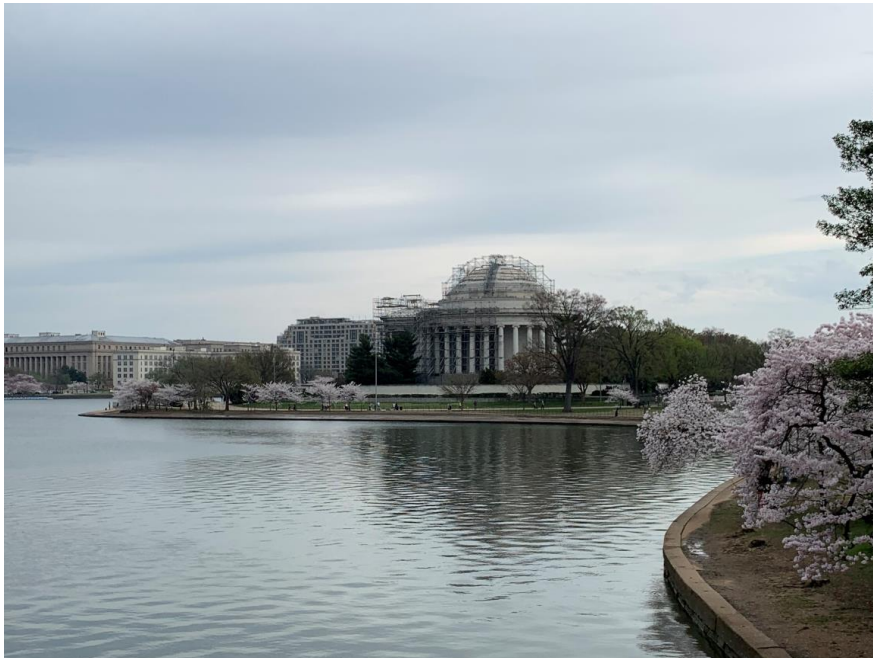
Asbestos Abatement at the Jefferson Memorial
