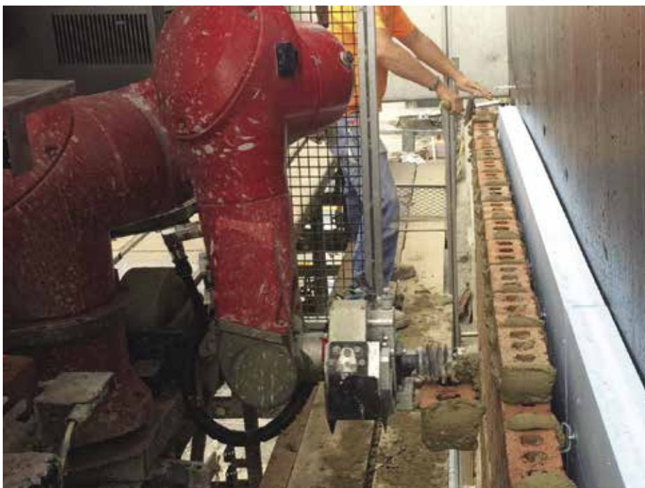
THE SAM ROBOT PARTNERS WITH A MASON TO LIFT EACH BRICK, ADD MORTAR AND LAY BRICKS INTO POSITION.
