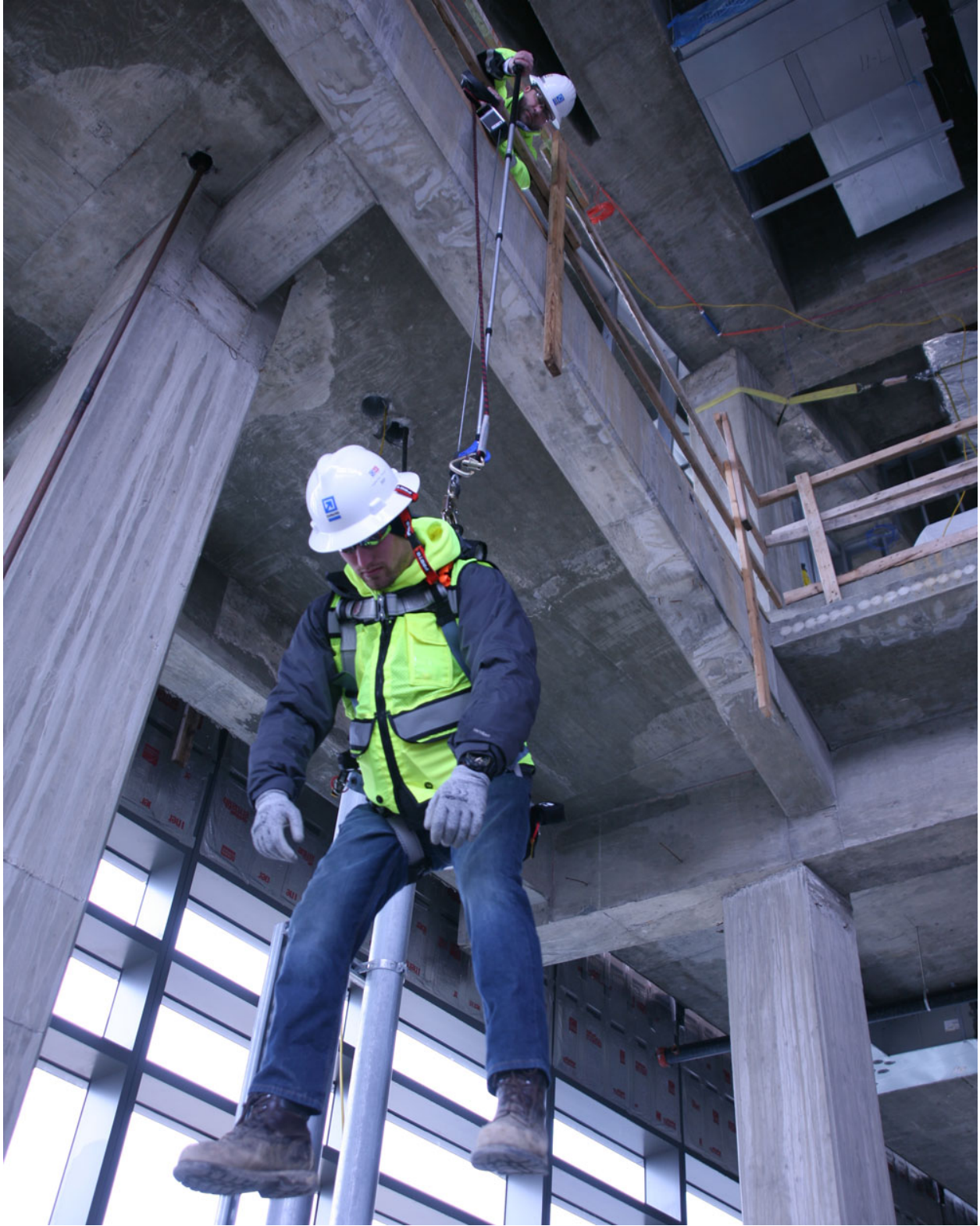
Checkmate Max 300R safety line being lowered to rescue mock-fall victim.
